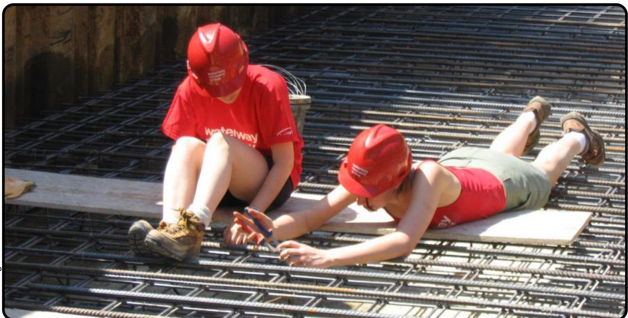
Assembling the reinforcing mesh for the final section of the base of the new Wey & Arun lock
